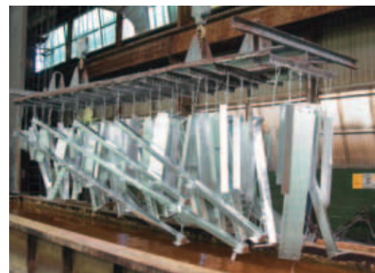
The Galvanising plant upgrade included the increase of our pickling capacity which is shown by the increase in the number of tanks in the photo. The product in the top picture is coming out of the caustic tank which degreases the product. The product is now ready to go into the rinse tank. The second picture shows a jig fully loaded with light structural work post Galvanising about to be quenched.
