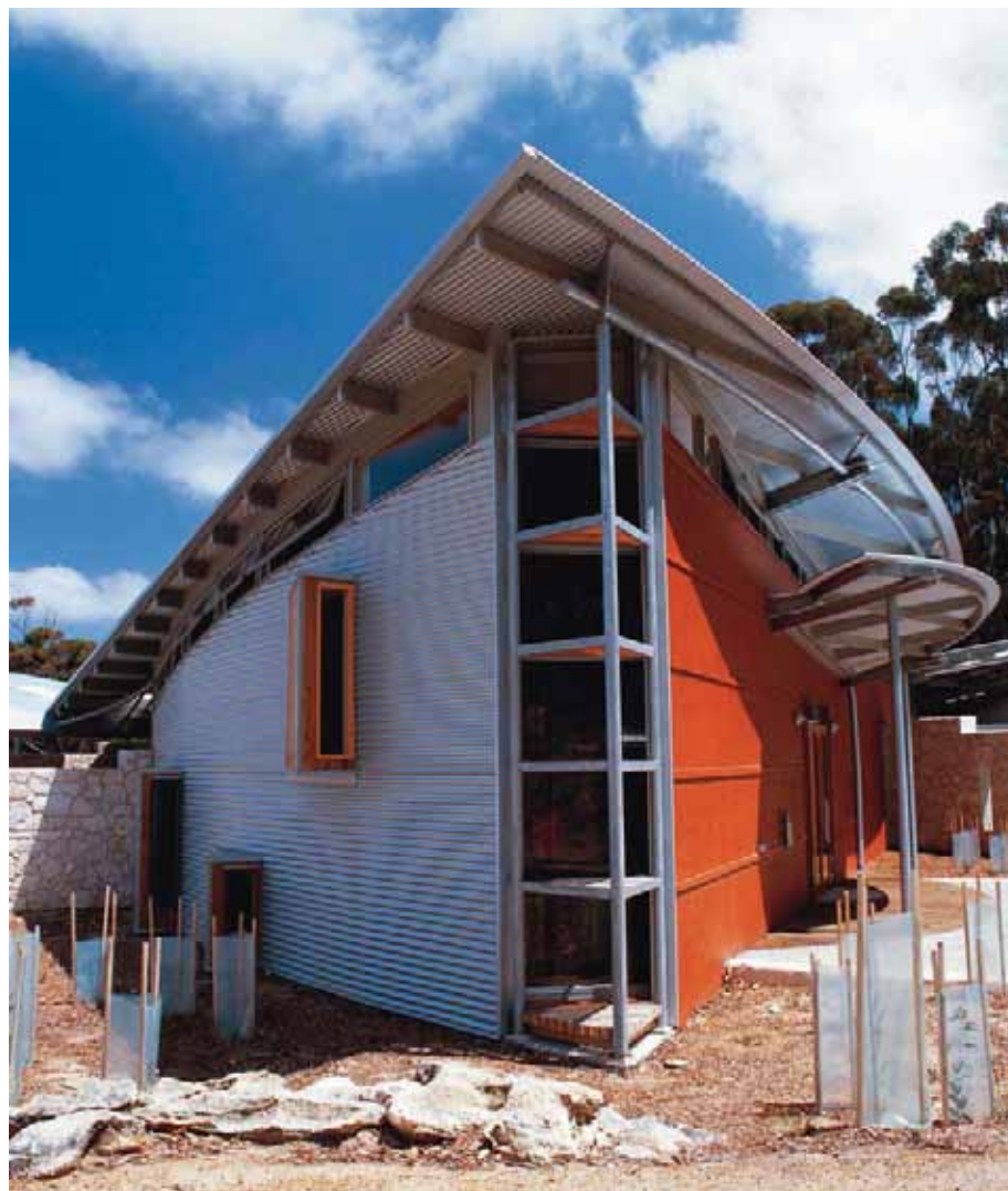
Galvanised steel in an architectural application.
