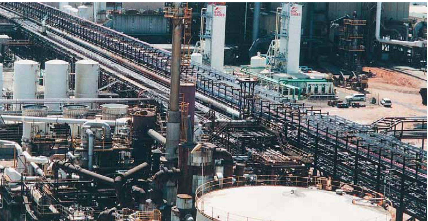
Ezustrut cable support system at a mining processing plant.
