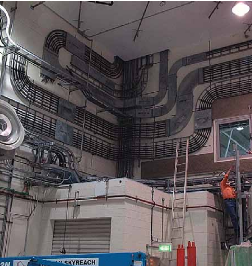
Ez Strut cable support systems in a manufacturing plant
