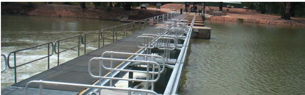
Galvanised steel works on a Murray River lock
